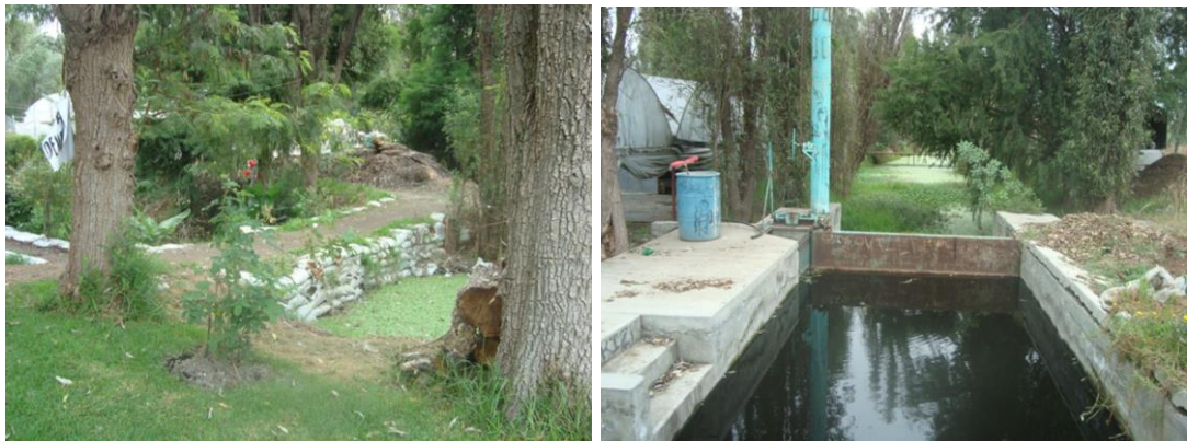
Figure 7.7 Locks to control the channels flow in San Luis Tlaxialtemalco.
