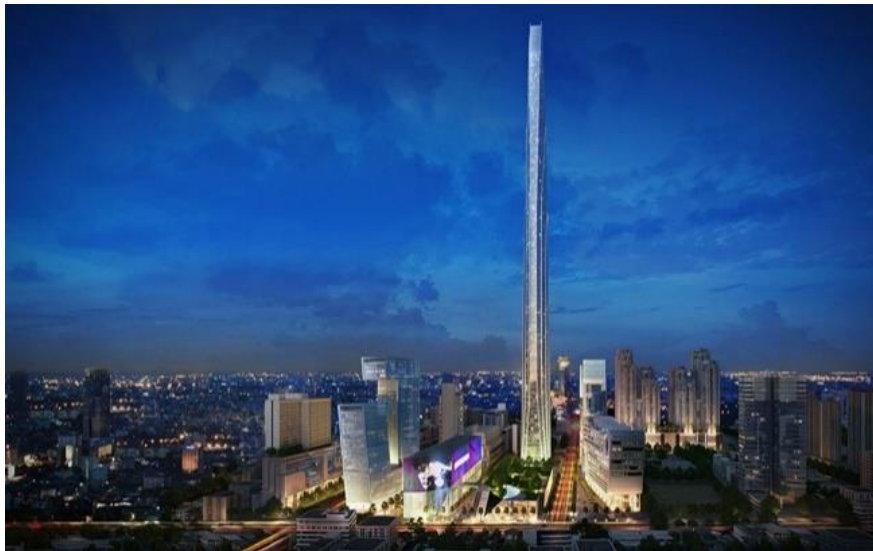
G Tower Grand Rama 9 Grand Canal Land LEED BD+C: Core and Shell v3 Registered in 2014; certification in progress
