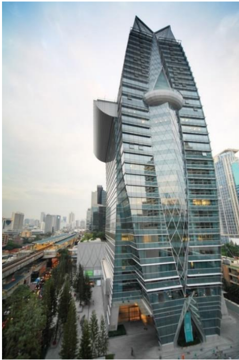
Park Ventures Ecoplex Univentures LEED BD+C: Core and Shell v3 Certified LEED Platinum in 2012
