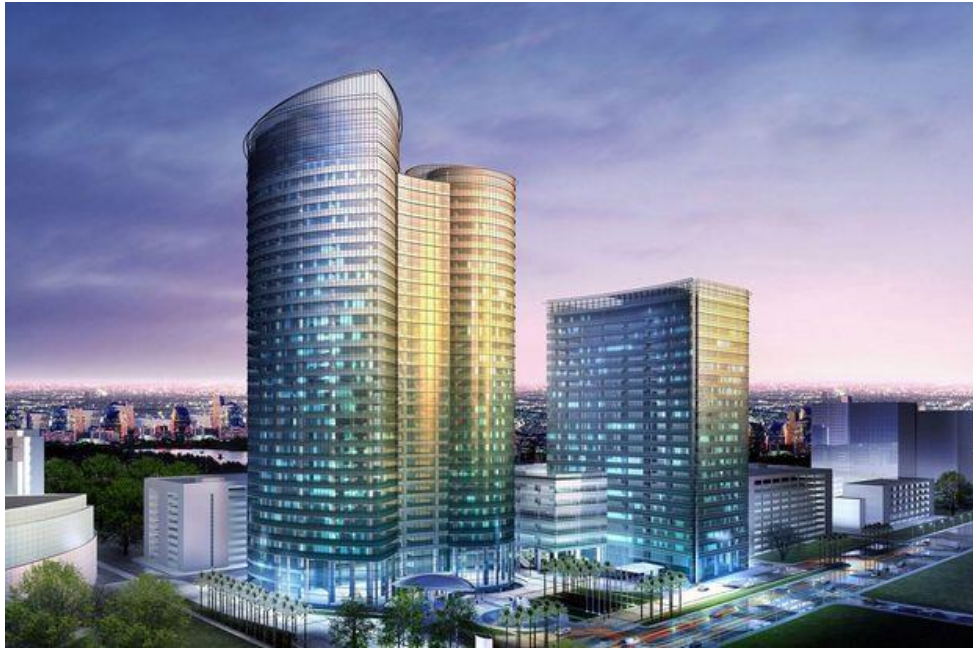
Figure 40 Energy Complex (EnCo) by PTT
