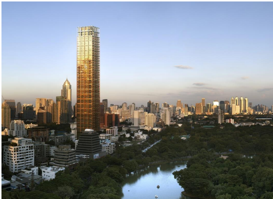
Figure 35 Nimit Langsuan by PACE Development Corporation
