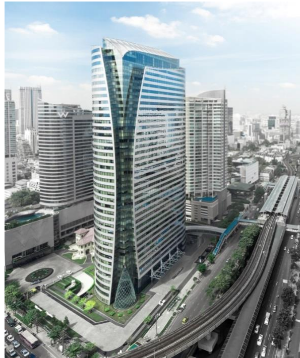
Sathorn Square Golden Land Property Development LEED BD+C: Core and Shell v3 Certified LEED Gold in 2013
