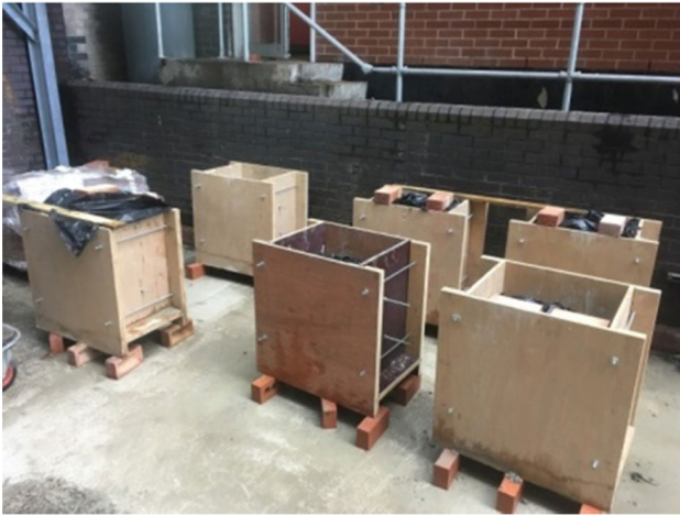
Fig. 1 Moulds for six kerbs at the casting stage
