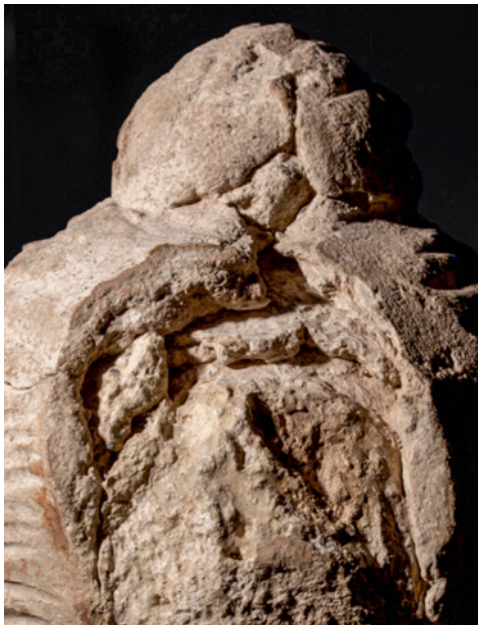
Fig. 3. Detail of the rear of the head, showing the inner stucco layers, irregularly applied on top of one another. These layers are composed of a lime-based stucco with some gypsum, large mineral aggregates (schist(?)) and vegetable fibres to counteract shrinkage upon setting. A finer, smoother layer of a similar composition, but with smaller aggregates, is applied atop the coarse layers and modelled while still fresh, as can be observed by the wide incision at the bottom left of the image. © G. Verri. Courtesy of Victoria and Albert Museum.
