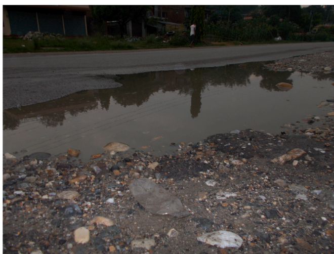
Fig. 4. Unclear edge of the road as potholes fill with water during the rainy season [P1, Grade 10, Boy].
