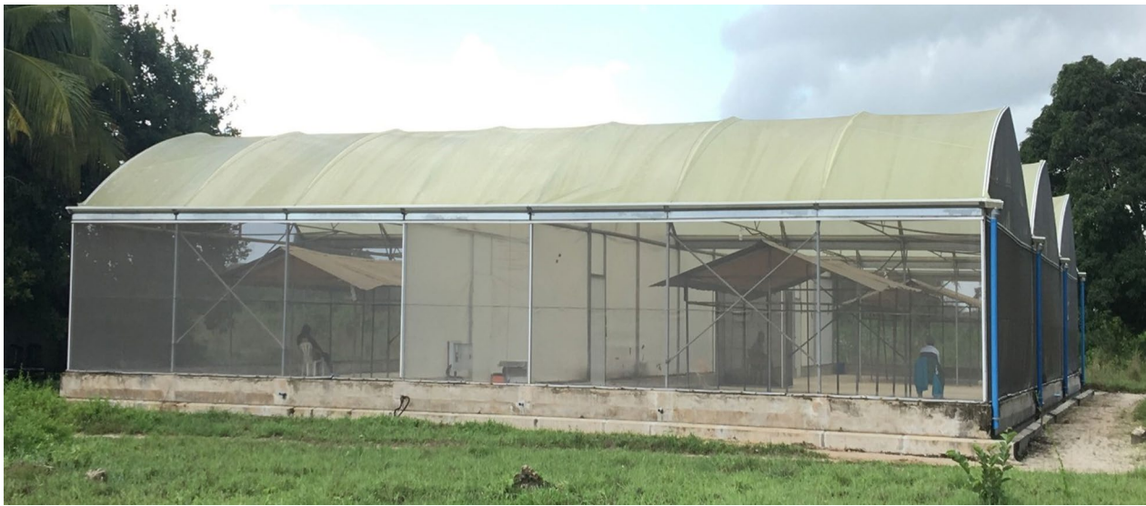
Fig. 1 A semi-field system (SFS). A semi-field system (SFS) with 29 × 21 m built from a fabricated greenhouse frame modified to make two chambers with a central corridor and an opaque polyethylene roof for rain protection
