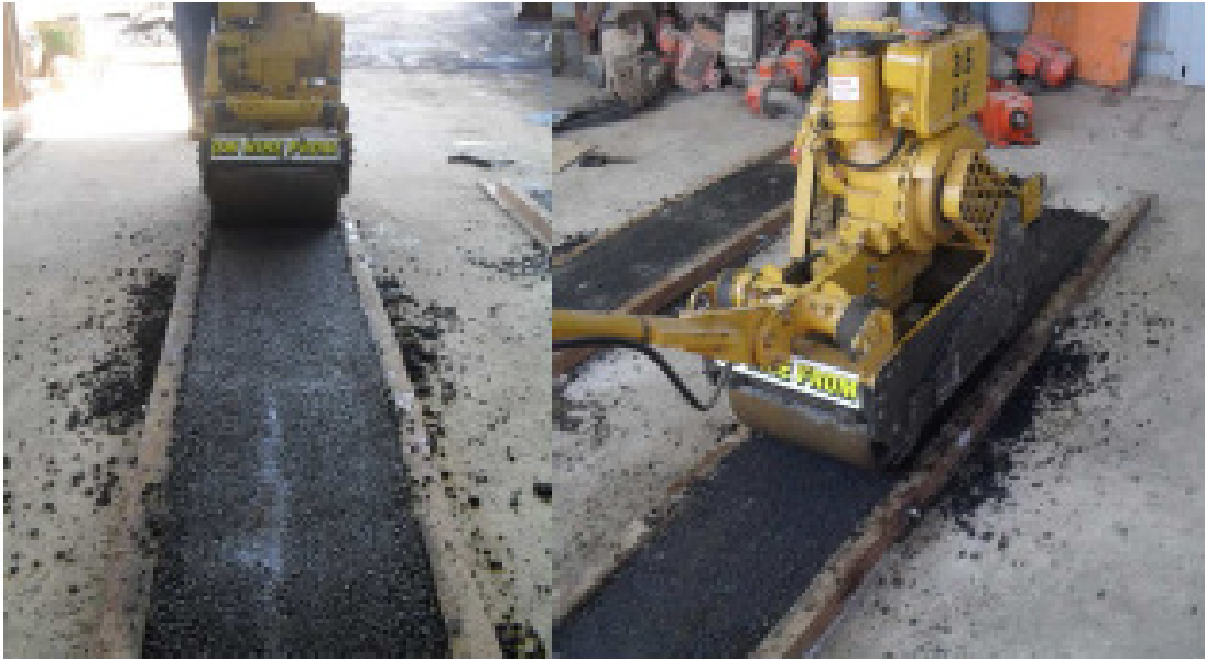
Figure 3.3 Photographs of the Compaction Process at the Plant (Mbaraga, 2011)
