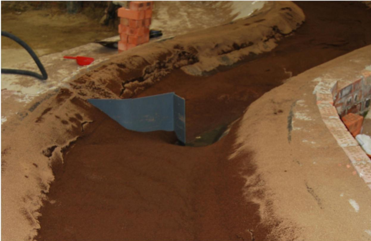
Figure A-34: Photo 1 of 60° structure with L-shaped attachment
