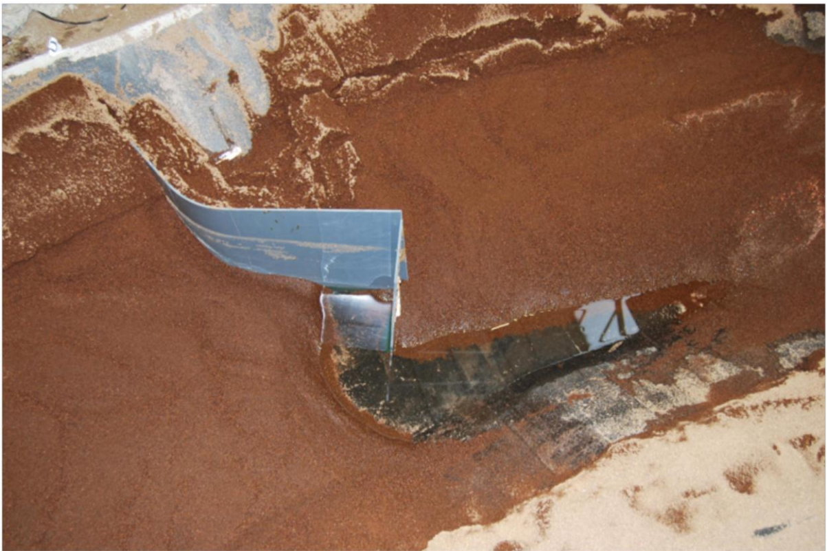
Figure A-27: Photo 4 of 45° structure with L-shaped attachment
