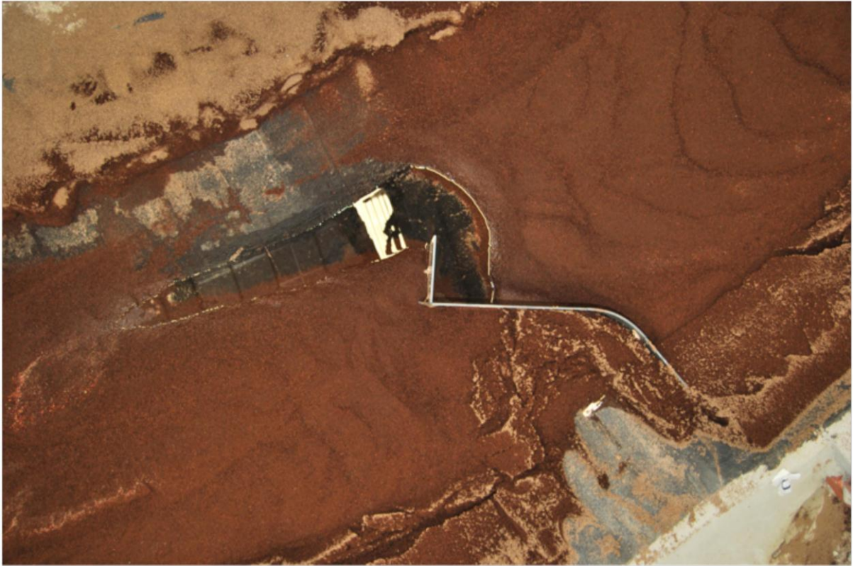
Figure A-26: Photo 3 of 45° structure with L-shaped attachment
