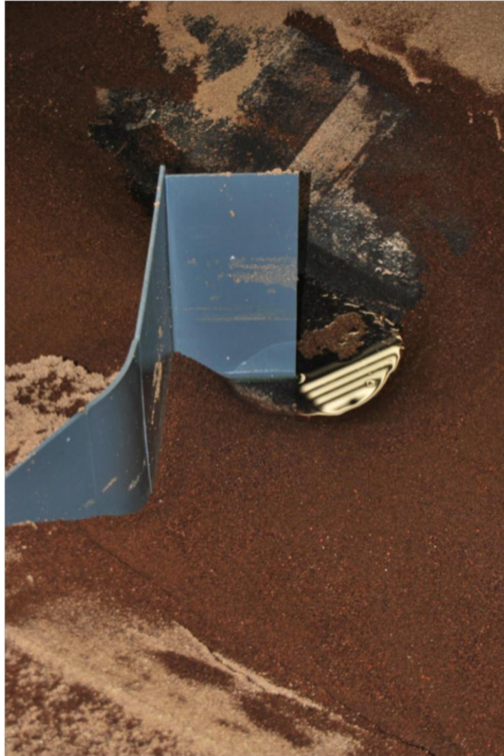
Figure A-38: Photo 5 of 60° structure with L-shaped attachment
