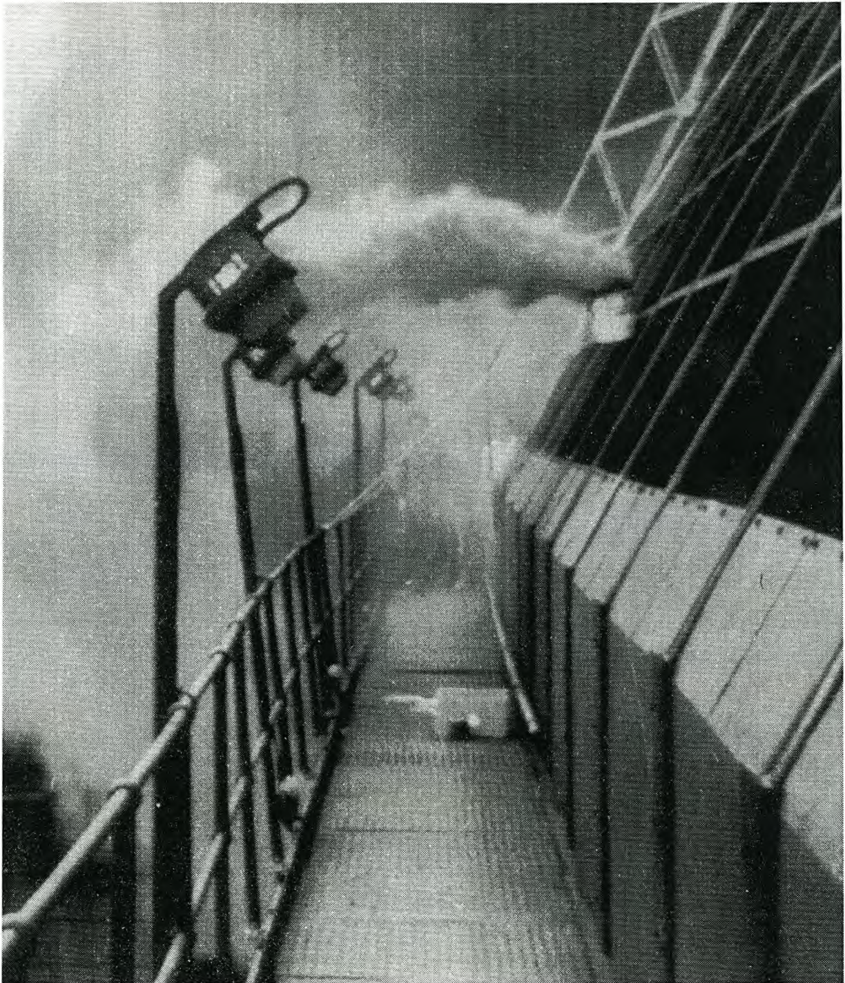
Fig. 8.4.6 Plume Air Recirculating in Air-Cooled Steam Condenser
