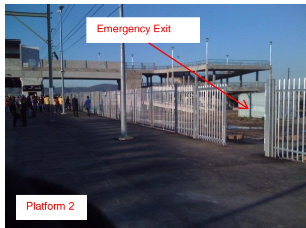
View of the side platform emergency exit gate
