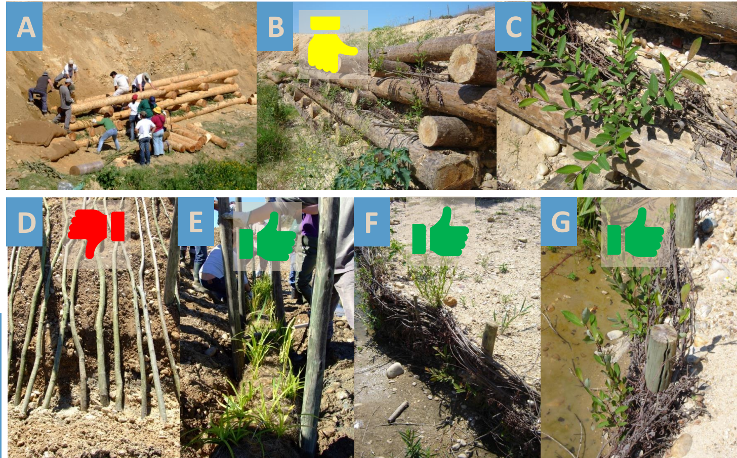
A, B e C: Cribwall D: Brush mattress E: planted coconut fiber rolls F: Wattle fences G: Live fascines
