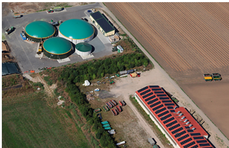
Figure 1: A typical biogas plant in our sample Source: (Überlandwerk Groß-Gerau GmbH, 2018)
