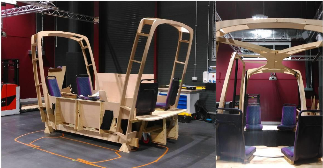
Figure 11.3 Construction of the Roof Structure
