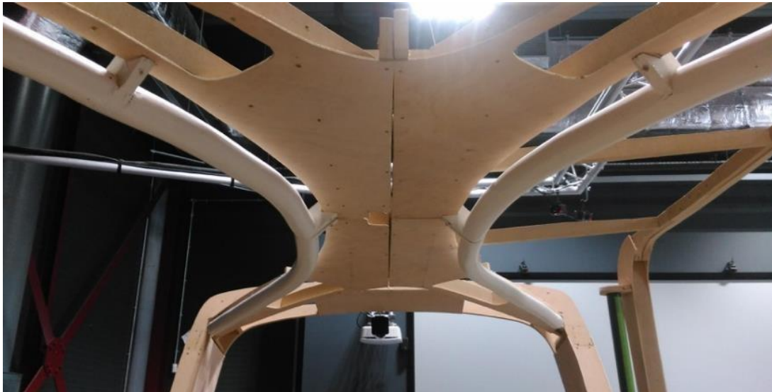
Figure 11.5 Handrails installed along the main Roof Structure
