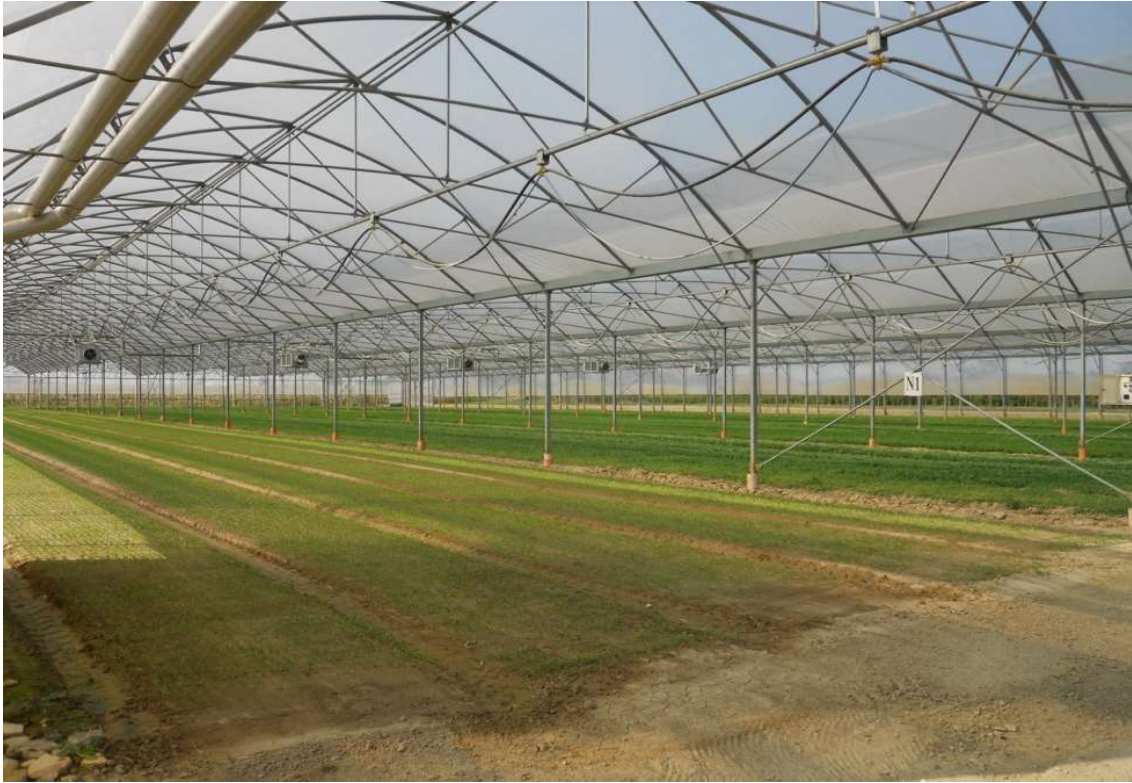
Figure 12. Glasshouse, with an area of 1 ha (10,000 m 2 ), employing a sandy substrate specific for growing these crops, ventilation and winter heating systems in place, with mechanical wings moving over the raised beds to irrigate, sow and harvest. Specialised cropping system of microgreens- in this picture: plants at different stages of growth. Farm location: Borgoricco, province of Padova, Veneto, Italy (07/09/2016).
