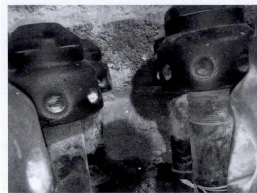
Fig. 3 Install dislocation of air cap [15]
