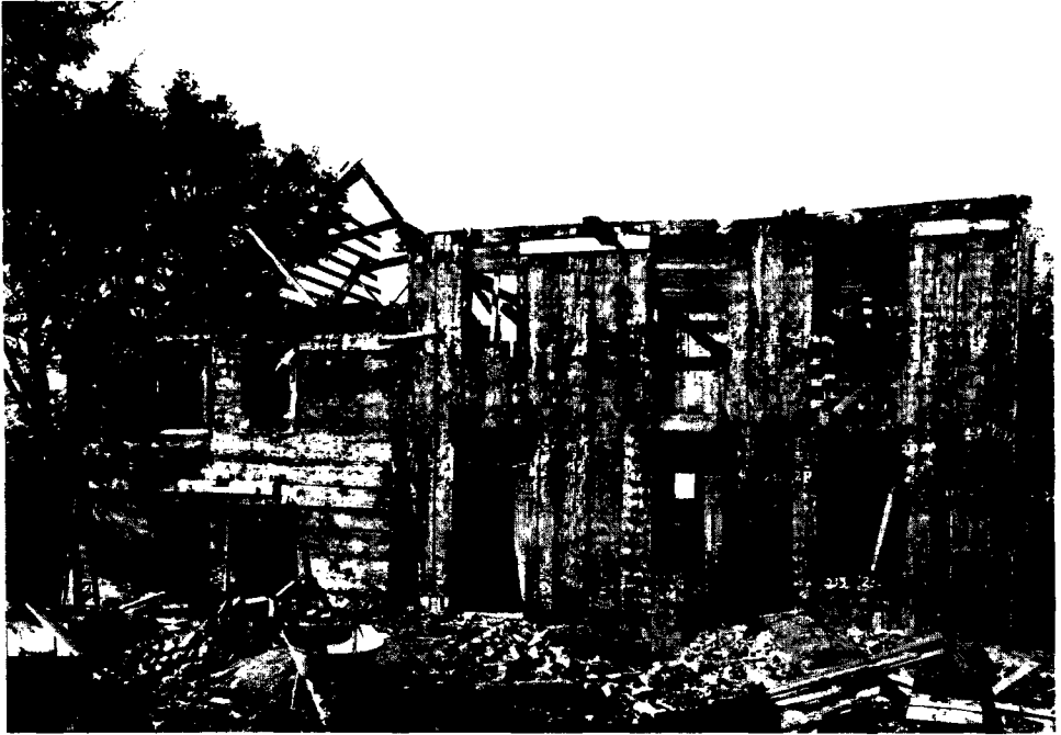
FIG. 7. SHELL OF THE MOTT HOUSE FROM THE EAST. The 1680 section at the left is sheathed with horizontal boards nailed to its vertical studs. The surviving portions of its original roof are visible at the top. To the right is the plank-framed 1725 section. There are no studs under the vertical boards. (Photograph by Jan Armor.)
