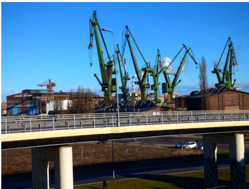
Figure 10. Newly constructed road in the former shipyard.
