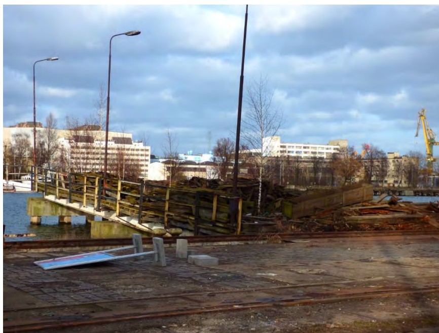
Figure 9. Ostrów Island over the canal.
