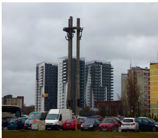
Figure 1. Newly constructed high apartment buildings on Wałowa Street.
