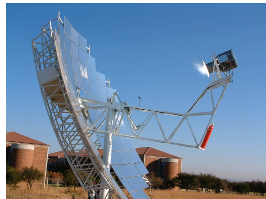
Figure 13: Eskom dish with Stirling generator 32
