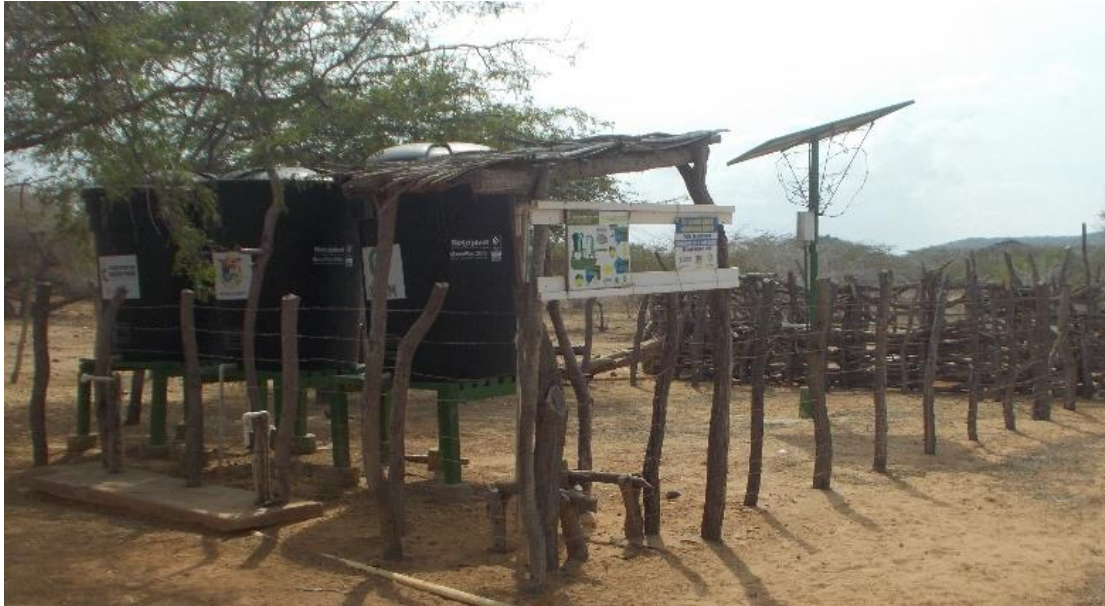
Figure 16. Punta Espada's damaged solar powered drilled well (May 2018)
