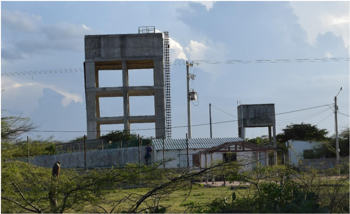
Figure 18. Mayapo's inoperative (left) and operative (right) elevated water tanks Source: Photograph taken by author
