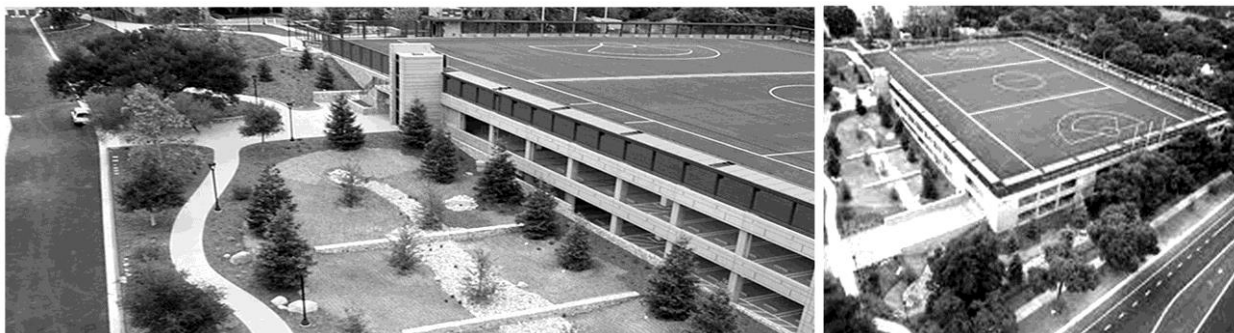
Fig. 8. Pomona College multi-storey car park, 2008, USA. General view
