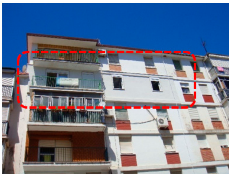
Figure 1. Building exterior view.
