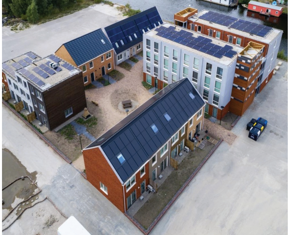
Figure 4.1 Loskade project in August 2019
