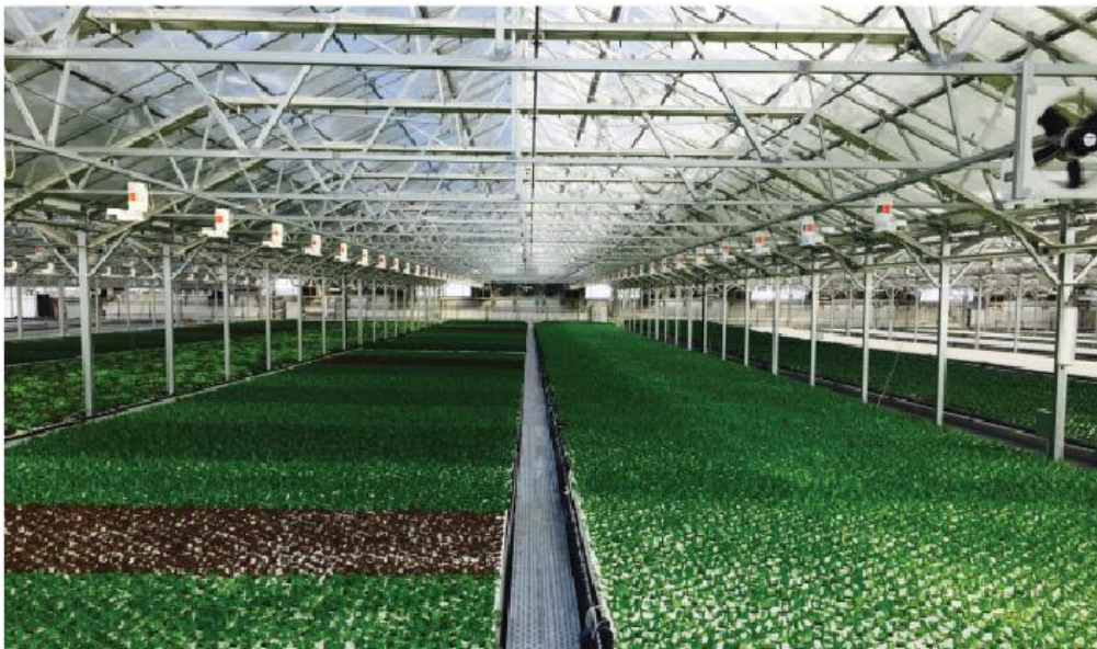
Figure 11 Gotham Greens Greenhouse Interior View, “Gotham Greens – Pullman” CNIGroup.org
