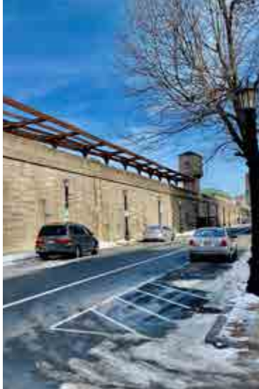
Union Station has one entrance on Lyman Street. The elevated tracks are supported by a massive granite wall.
