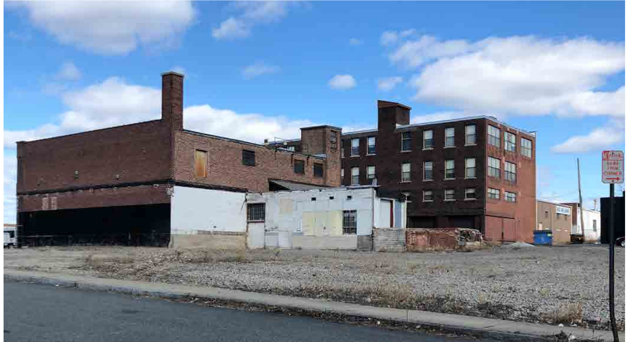
Vacant lots and distressed buildings on Alert Street and Fairbank Place provide opportunities for creative adaptive reuse.
