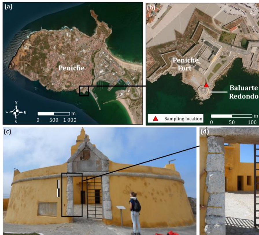
Figure S9: (a) Location of the AF05. (b) Location of Baluarte Redondo fort (Maps built with Esri© ArcMapTM 10.4, source of the satellite images: Esri, Digital Globe, GeoEye, i-cubed, USDA, USGS, AEX, Getmapping, Aerogrid, IGN, IGP, swisstopo, and the GIS User Community). (c) Main door (vertical scale 1m). (d) Surface used in lichen cover measurements (vertical scale 1.2m, horizontal scale 0.2m).
