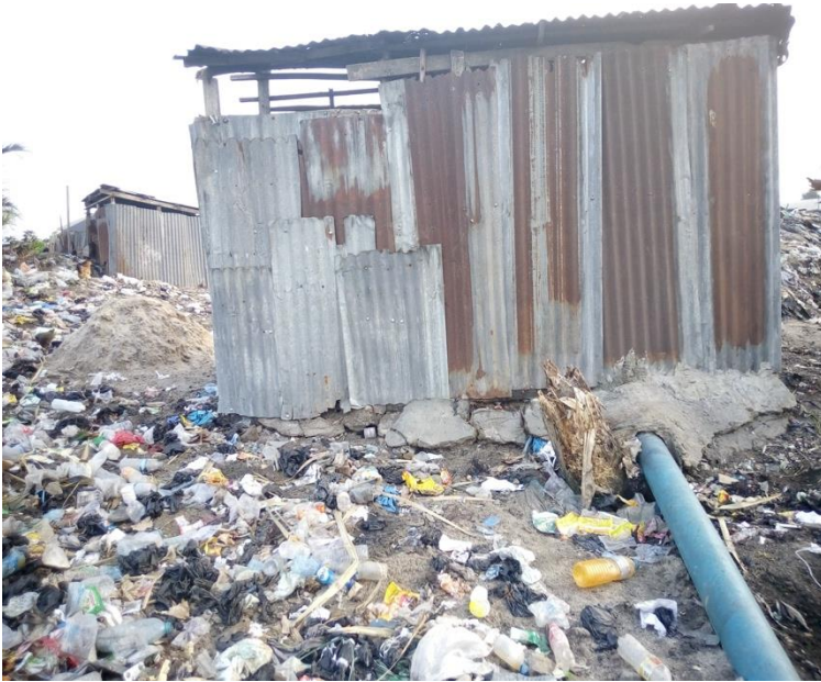
Plate 1. Latrine with a pipe emptying into a drain
