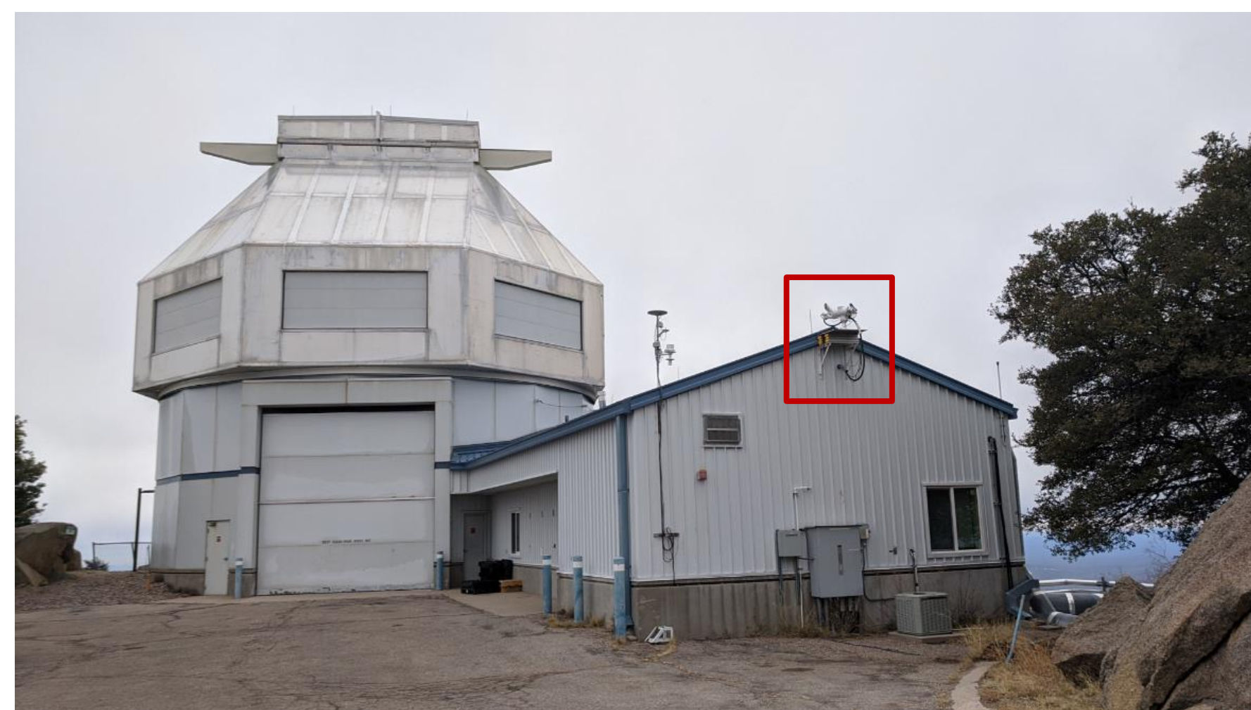
Fig. 2: The solar feed (red box) installed on the control building of the WIYN 3.5m. This location permits an unobstructed view of the sky above airmass 2 throughout the year and is accessible for periodic maintenance.
