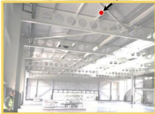
On-site visit showing beams specifications.
