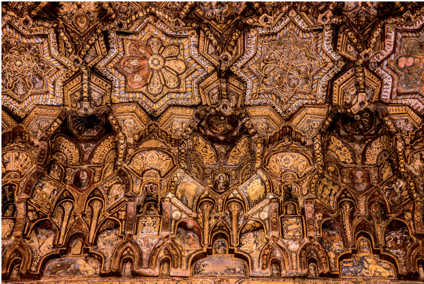
Fig. 2. The muqarnas ceiling in the 10th century Cappella Palatina in Sicily (photo: Idries Trevathan 2014).
