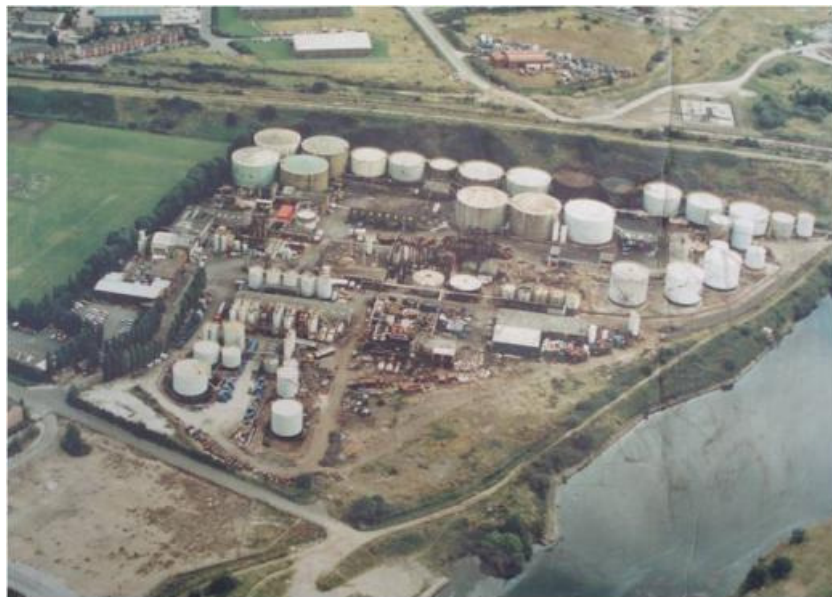
Figure 9.13: Cadishead Chemical Works, Salford, prior to remediation Developer/Remediation: Harrow Estates.
