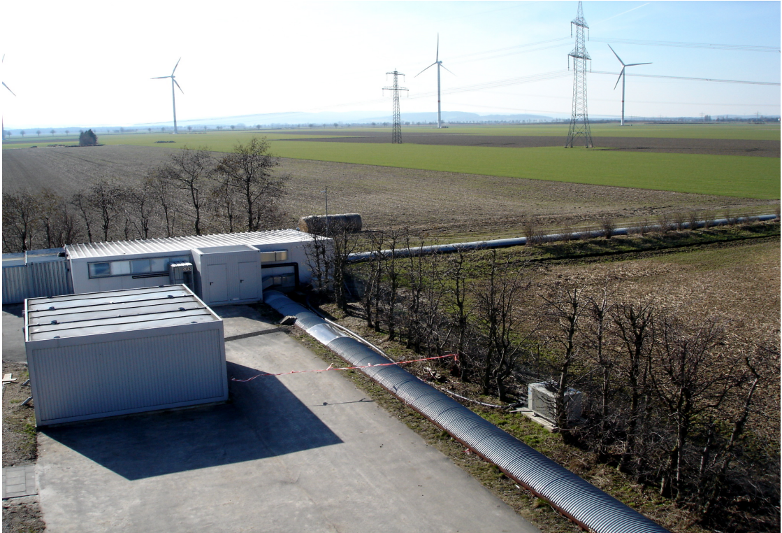
Figure 1.7: The GEO600 interferometric gravitational wave detector, situated in Ruthe, near Hannover, Germany. The two perpendicular 600 m long arms can be seen, meeting in the central station which houses the input laser, beam-splitter, and other optics and control electronics.
