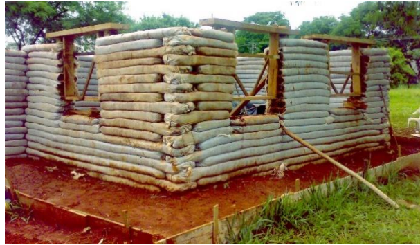
Figure 12. Construction of self-supporting orthogonal earthbag building.
