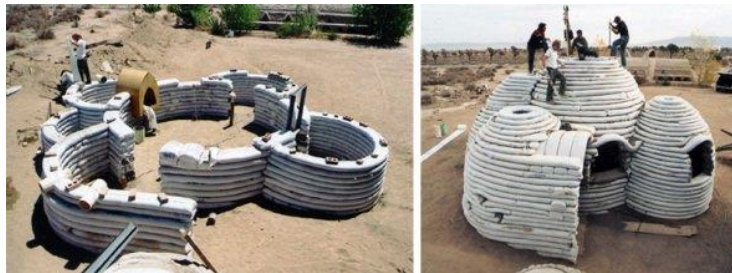
Figure 10. constructions of self-supporting SuperAdobe domes.
