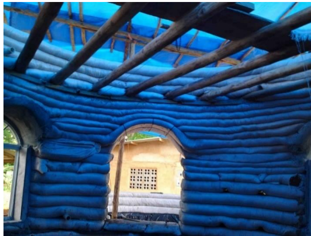
Figure 6. Construction of 2nd floor of Majestic Dome, Panamá.
