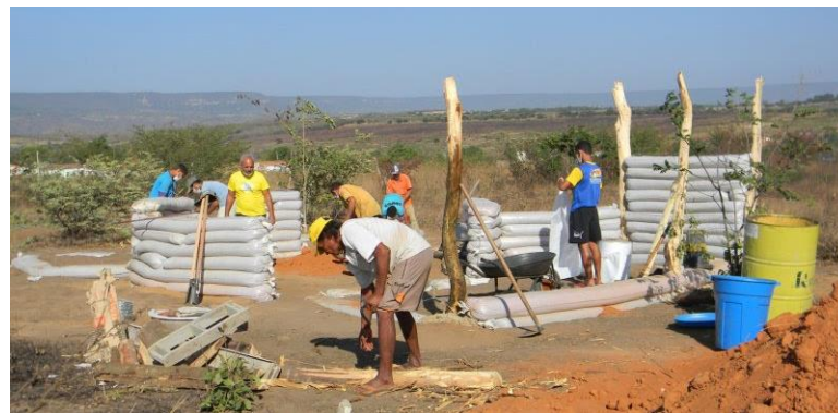
Figure 13. SuperAdobe construction with timber structure in Ceará, Brazil.
