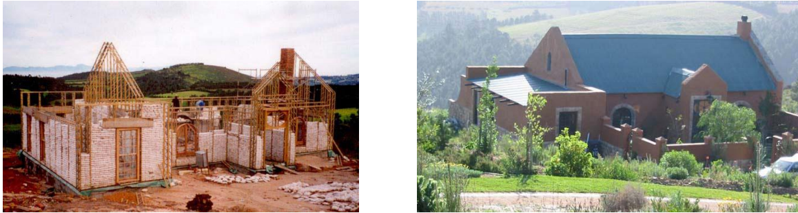
Figure 14. Before and after of a sandbag construction with Ecobeam construction
