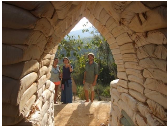
Figure 11. SuperAdobe gothic arch as a small entrance corridor.
