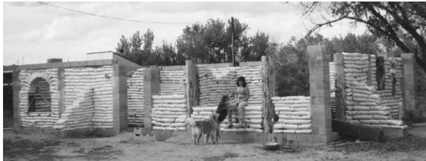
Figure 17. SuperAdobe construction made with precast concrete in Moab, Utah.
