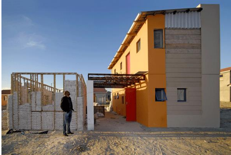
Figure 15. Housing buildings with one block under construction and other already done.
