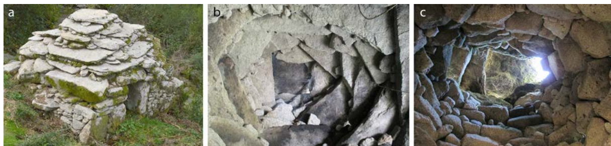
Figure 9 - a and b - external and internal views of a corbelled dome built with large-size plate shape granite units; c - internal view of a corbelled dome built with irregular plate shape granite units [1]. (“ branda ” of Gêmea).
