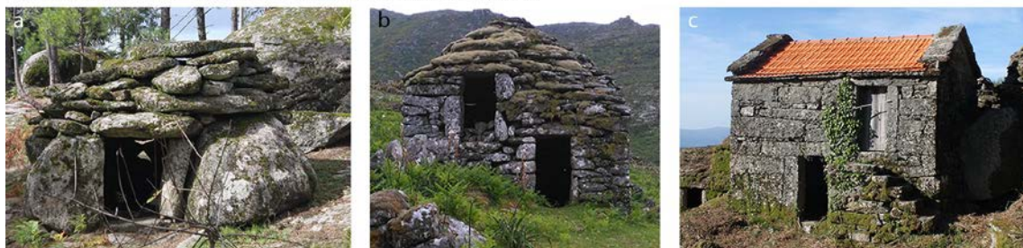
Figure 5 - Schematic examples of corbelled domes buildings morphological and typological main features, based in the “brandas” de Padrão study cases [1]. Examples of: a - single-storey shelter (“branda” of Travanca); b - two-storey shelter (“branda” of Rio Côvo); c - two-storey “branda” house (“branda” of Gêmea).
