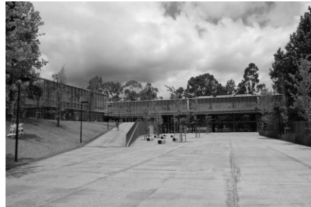
Fig. 4 Complete transformation of the school image. Escola Secundária de Lousada, Architect José Manuel Carvalho Araújo (2012) © André Santos
