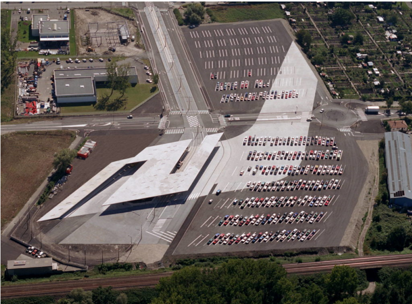
43. Car Park and Terminus Hoenheim North
