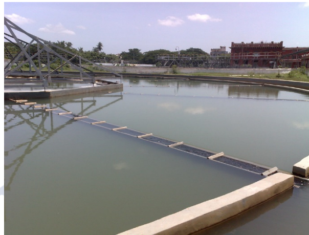
Figure I.3. Picture of a sedimentation tank employed during primary treatment ( Picture from Touzeen Hussain (2007) on flickr.com gallery )
