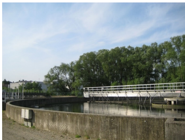
Figure I.4. Secondary wastewater clarifier (picture from Annabel (2011) Wikimedia Commons)
