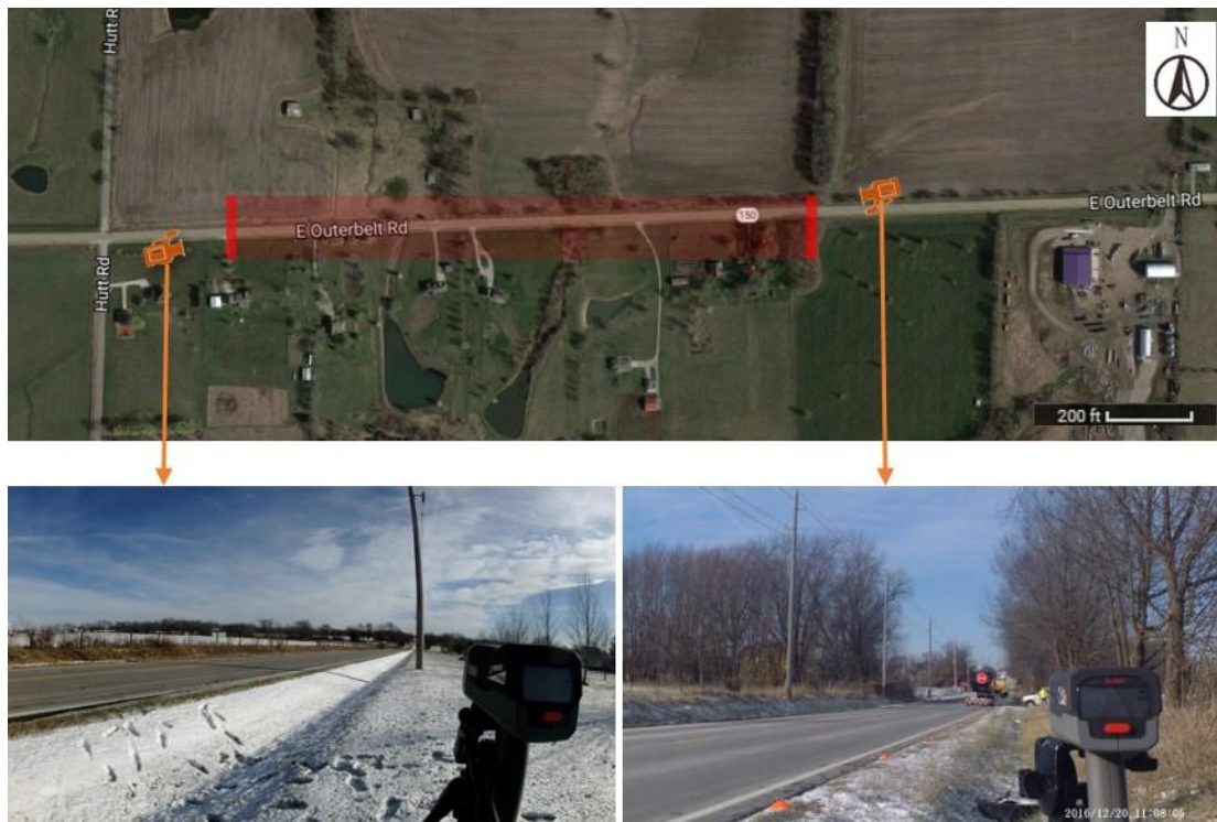
Figure 4.1.1.3 Field Settings on MO-150 Highway Work Zone (Google Maps 2017)
