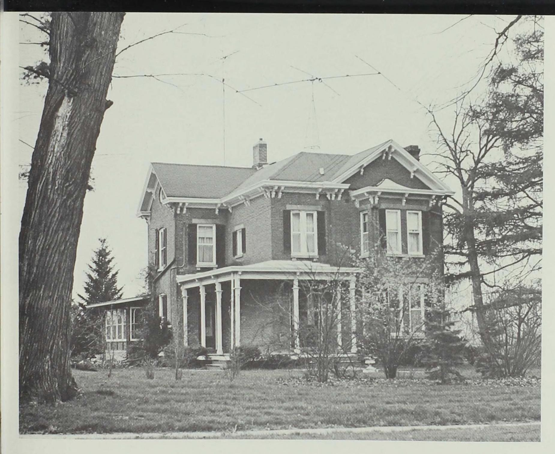
the early houses generally had steep roofs with gables that formed right triangles, permitting the use of the top story for bedrooms or attic space. The low-pitched roofs in Iowa, which sacrifice space that could have been added at little extra cost or labor, may reflect the hazards of high winds.
