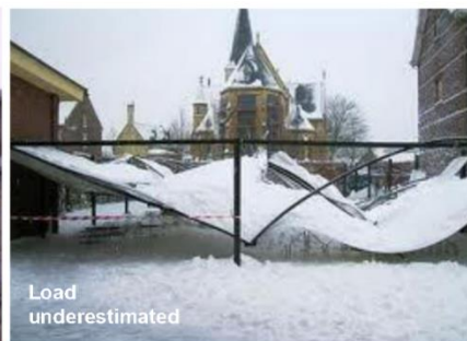
Roof collapse (2012/13)
