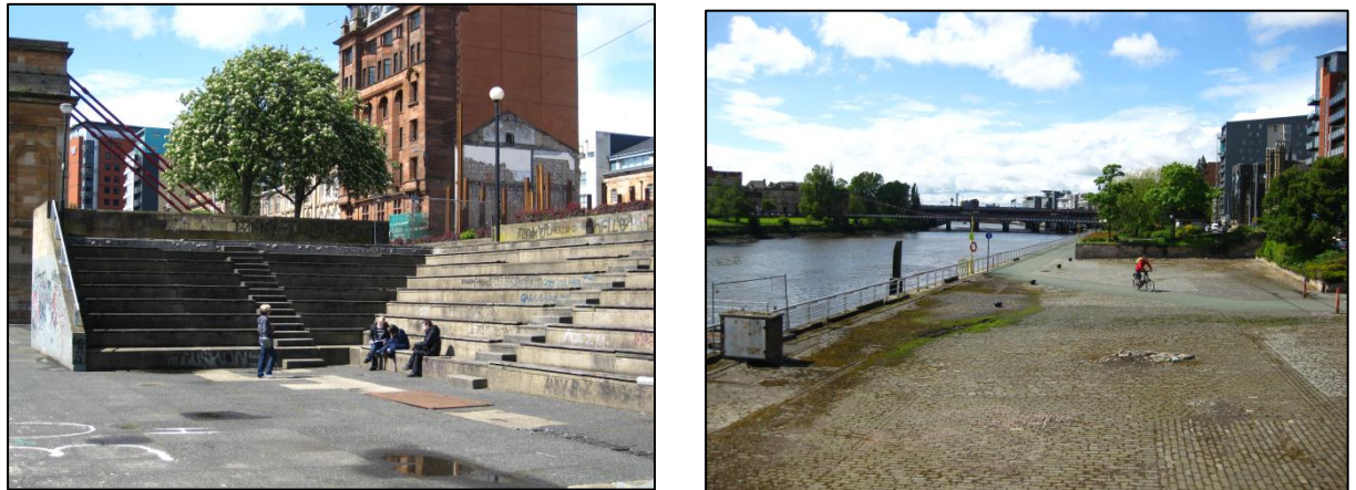
Figure 9.4 Custom House Quay today still awaiting redevelopment
