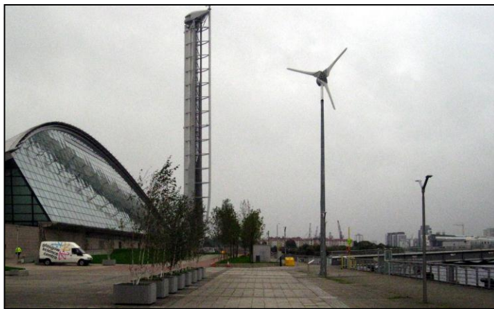
Figure 7.24 The wind turbine at Pacific Quay – the only opportunity for active engagement and discovery
