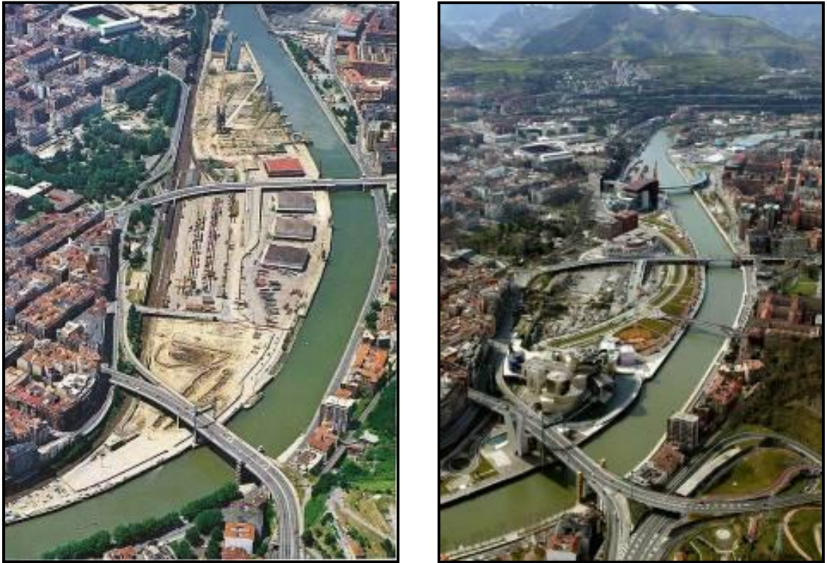
Figure 6.3 The Abandoibarra project (left – 1992; right – 2005); an example of a regenerated waterfront and the resultant new public places (Source: www.skyscrapercity.com )
