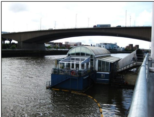
Figure 9.10 'The Ferry' river venue, the only existing boat restaurant on the Clyde today (behind it, view of Kingston Bridge)
