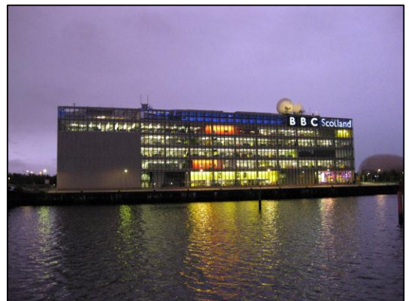
Figure 7.13 The BBC building (view South from the opposite river bank)
