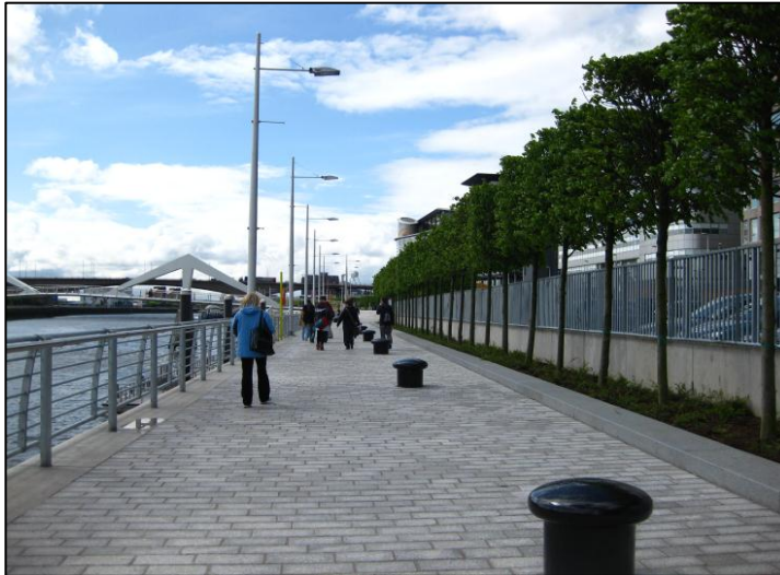
A. The area of the new public place between the Riverboat Casino and the river
