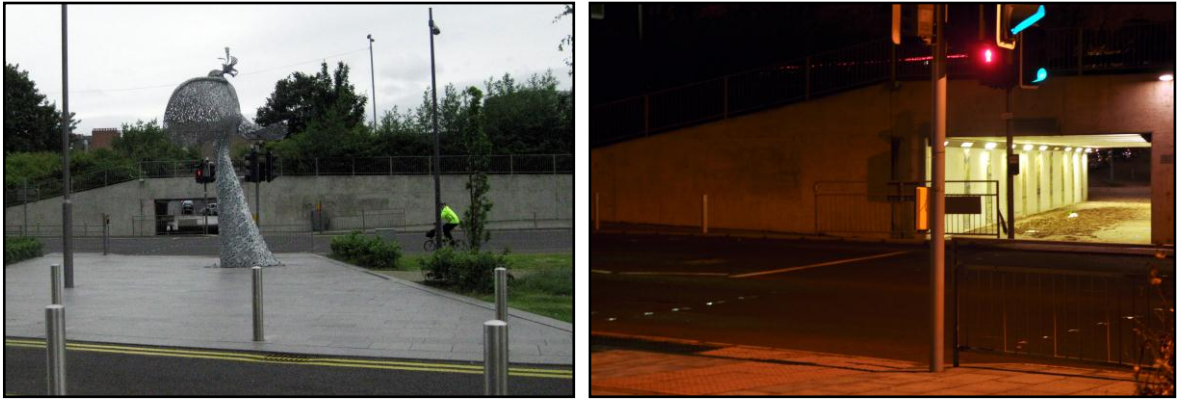
Figure 8.20 The Meadow Road Underpass (day and night time)
