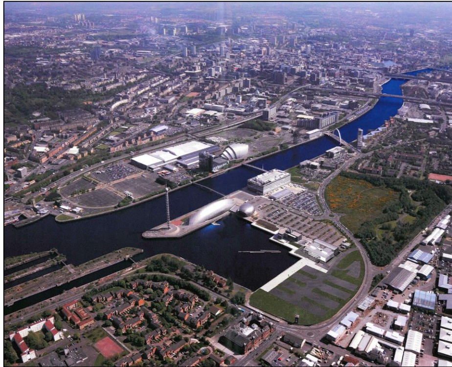
Figure 7.17 Aerial view of the Pacific Quay site today (Source: courtesy of Scottish Enterprise)
