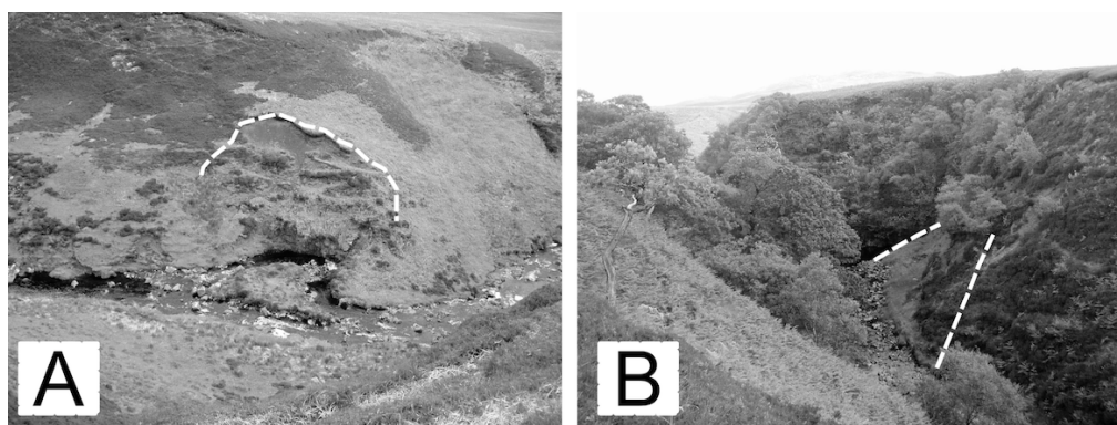
Figure 6.6: The photograph on the right correspond to stream 38 where glacial material is being supplied to the rivers from unstable slopes, the scar of the landslide is marked with the white dashed line. On the left, a small talus cone (right bank of the picture, white dashed line) located downstream of the 13.6 ka knickpoint of stream 25. Note the steep valley walls of the picture of the left.
