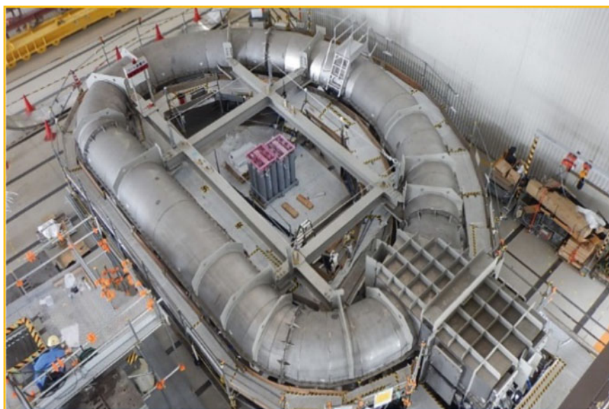
Fig. 26.5 Poloidal field coils
