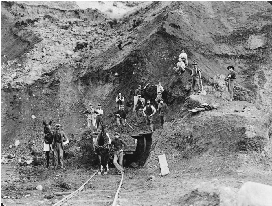
Figure 1: Man-power. Railway construction workers pictured at their work-site about 1910 (location unknown). The basics of tools and equipment reminded the same - shovels and carts for moving tonnes of earth to create the flattest course for the rail-line. Photograph. Railway Construction Workers . Making New Zealand: Negatives and prints from the Making New Zealand Centennial collection. Alexander Turnbull Library, Wellington, Ref: PAColl-3060-016.. /records/23108227
