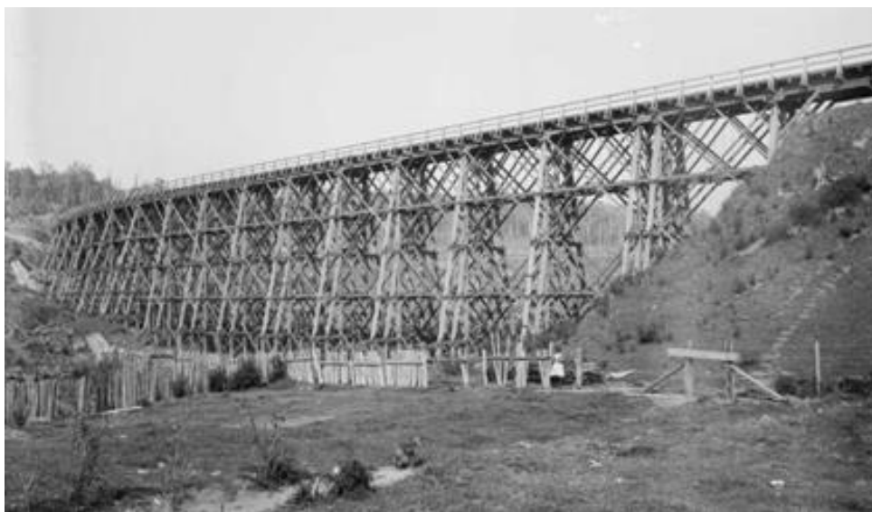
Figure 23: Viaducts such as this one at Ormondville required specialist workers to complete the engineers' design. Photograph. Hawke's Bay's Ormondville viaduct . Alexander Turnbull Library, Wellington, Ref: 1/1-025507-G. /records/23201446
