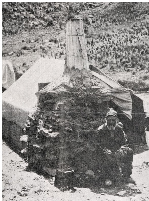
Figure 18: The Otago Witness titled this photograph 'The Original Navy.' Single men lived in smaller tents, often shared with another worker. The essential fireplace provided warmth and light to the simple accommodations on the Otago Central line. The sod construction gives an air of permanence that a wooden chimney lacks. Photograph. "The Original Navy", Otago Witness , 18 Sep1901, 39. Hocken Collections - Uare Taoka o Hākena, University of Otago, S19-228a
