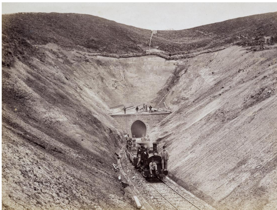
Figure 14: Men at work on a tunnel on the Chain Hills line south of Dunedin. The photograph shows an enormous amount of earth and vegetation has been cleared in the approach for the tunnel. Photograph. Chain Hills tunnel, south end , n.d. Hocken Collections - Uare Taoka o Hākena, University of Otago.
