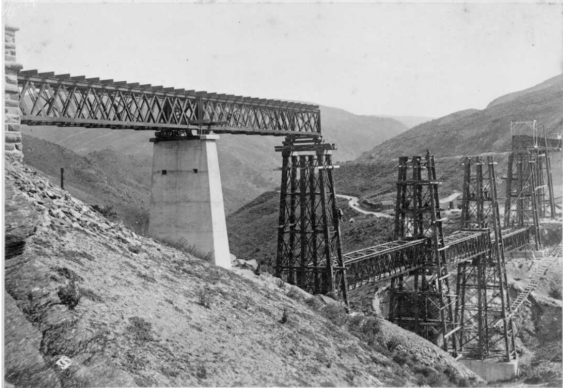
Figure 25: Wingatui Viaduct spanning Mullocky Gully. Opened in 1887 it was the largest in New Zealand, and they speculated, in the southern hemisphere. All the material was manufactured in Dunedin or on site. It was 690 feet long, and 154 feet eight inches from bridge to creek bed. The main girders were raised by specially built hydraulic presses. Several speakers at the opening noted that it had taken longer than expected to reach this point (eight years since the line began in Mosgiel). The engineer, inspectors and contractor were praised for their work. 269 Photograph. Wingatui Viaduct under construction, on the Otago Central Railway Line [photographer unknown], circa 1888, Alexander Turnbull Library, Wellington, Ref: APG-1190-1/2-F.. /records/22605789
