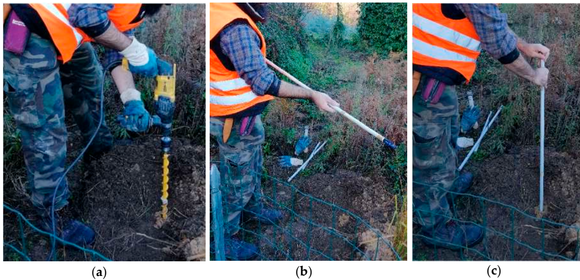
Figure 9. Vertical installation: (a) Creation of the vertical hole; (b) Positioning of the WaterScout in the PVC pipe; (c) Insertion of the sensor in the hole.
