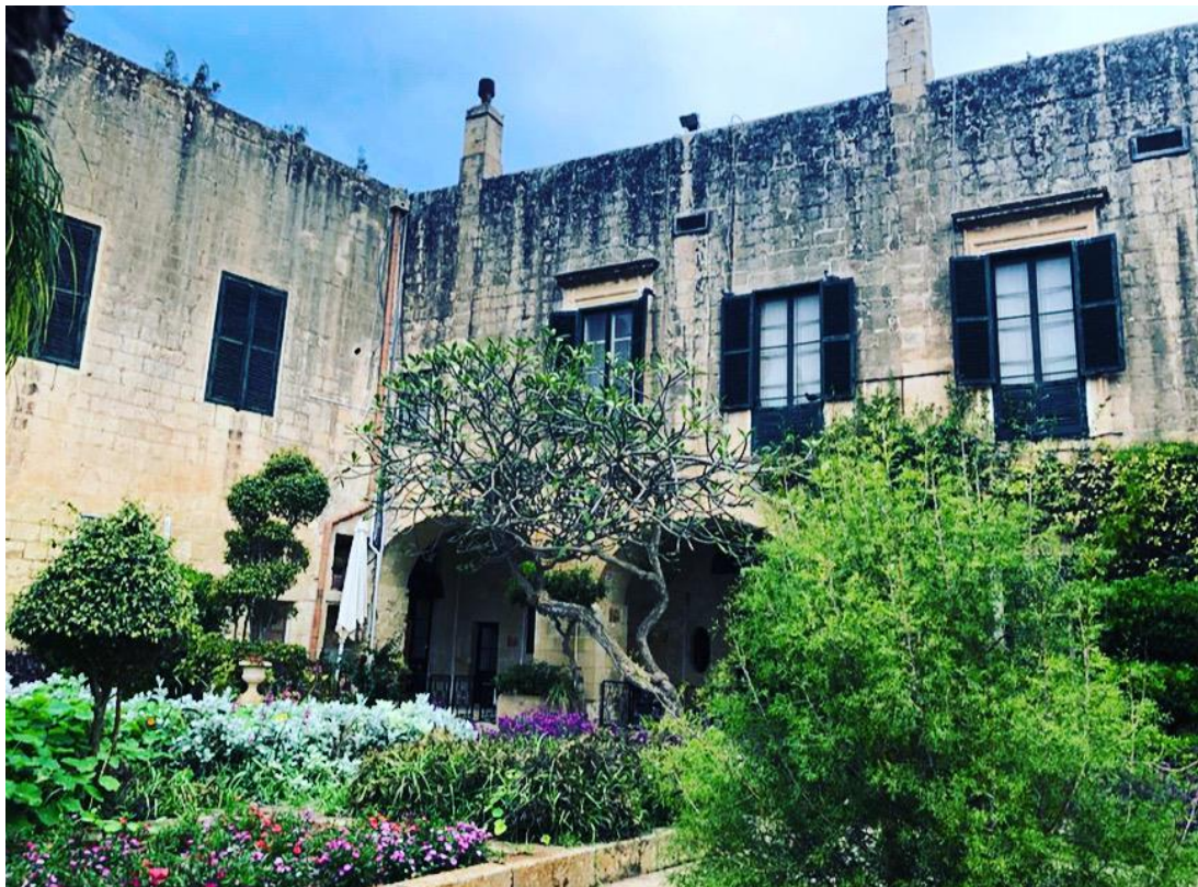
Figure 3.8: A loggia, timber louvered apertures, thick walls and lush vegetation comprise some of the passive environmental design strategies inherent to San Anton Palace, Malta (Source: A Wismayer)
