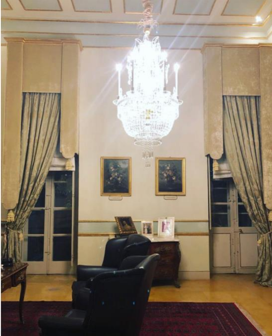
Figure 5.9: Heavy, fixed curtains compromise the potential for environmental control, San Anton Palace (Source: A Wismayer)
