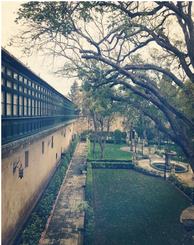
Figure 5.5: West-facing timber balcony overlooking the private gardens, San Anton Palace (Source: A Wismayer)
