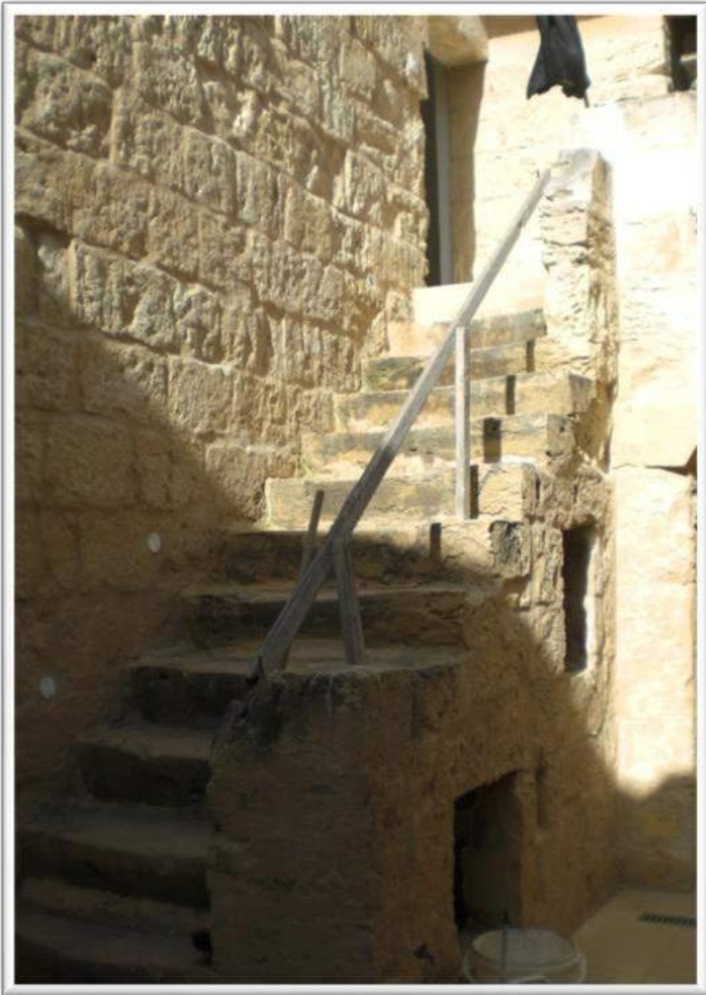
Figure 4.5: Staircase in courtyard providing externalised access to the first floor (Wismayer, 2013)
