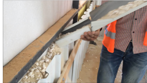
(d) Thermal mass by cavity fill (ID 3; 60 mm sand and gravel mix in wall cavity)
