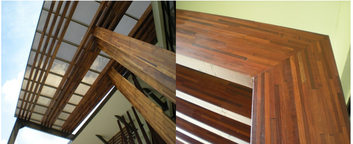
Fig. 2.3 Glue laminated timber in existing timber structure
