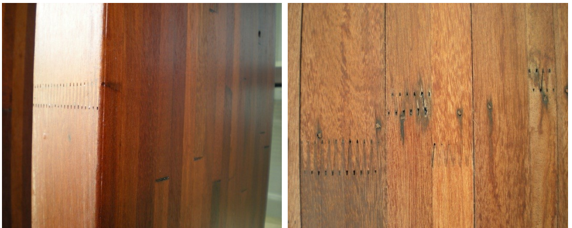
Fig. 2.4. Finger joints of glulam which can be in horizontal or vertical arrangement
