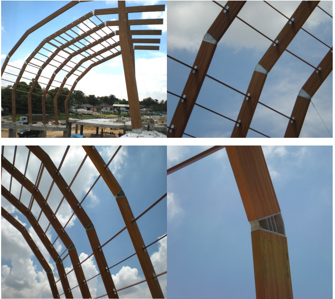
Fig. 4.7. Close up of bonded-in connection
