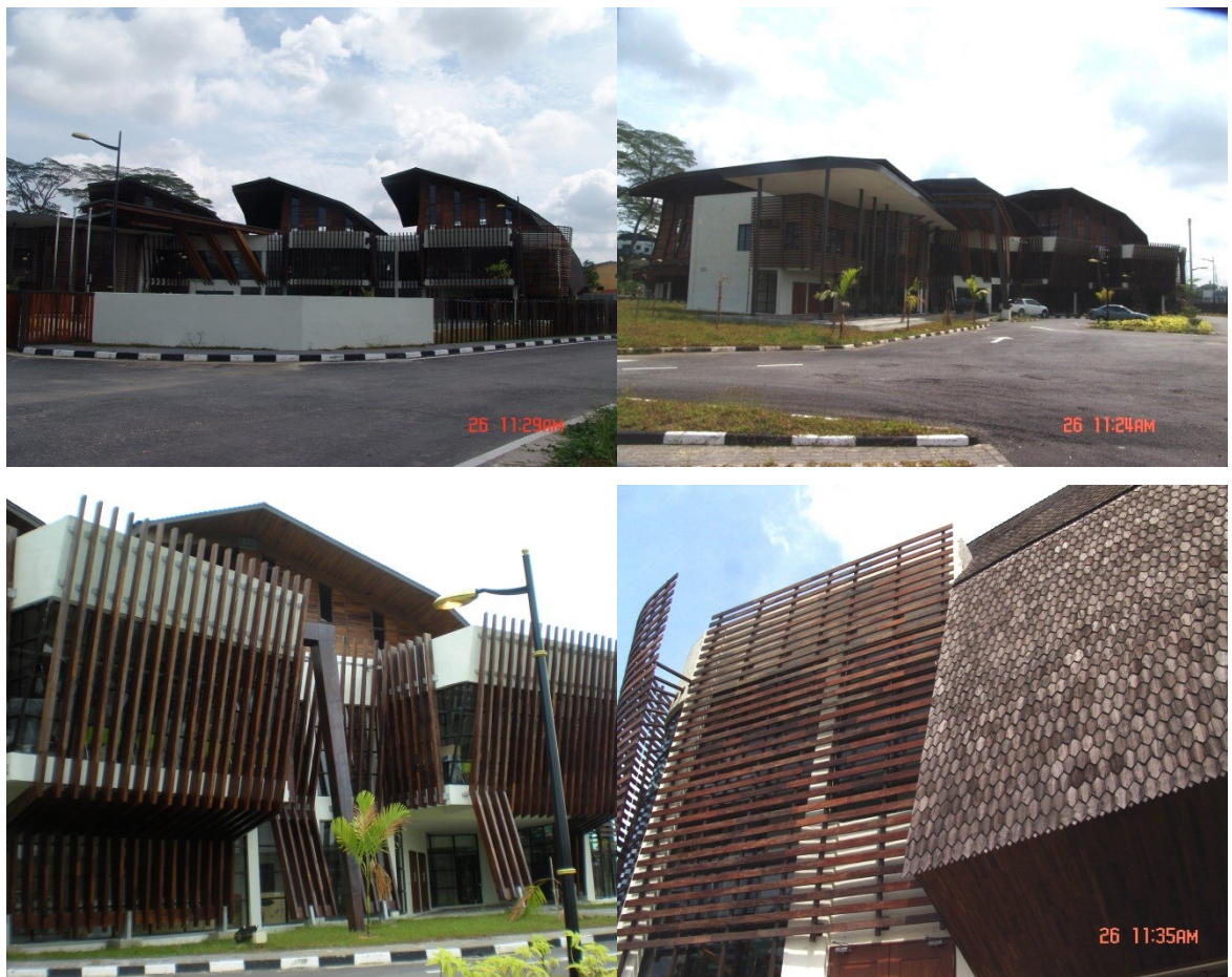
Fig. 4.4. Malaysian Timber Industrial Board (MTIB) exhibition hall in Johor
