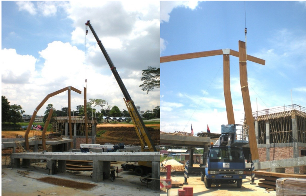
Fig. 4.8. A crane lifting a section of the arch
