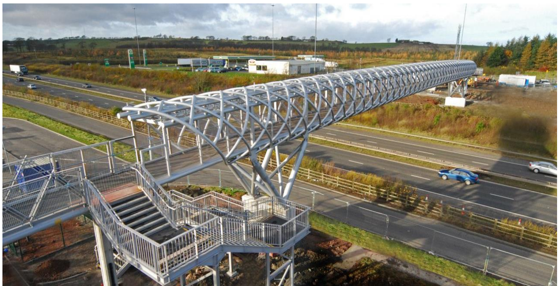
Figure 2.2 The M8 Harthill Footbridge constructed in a steel truss structure in Lanarkshire (SH Structures, 2018)
