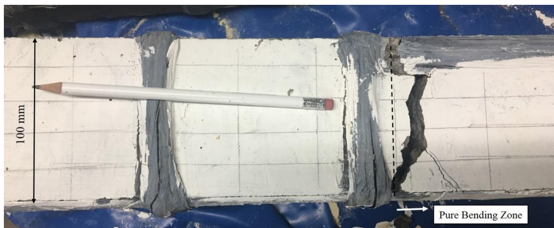
Figure 5.11 Crack and failure of the over-reinforced and seawater-exposed Beam CC2.2-S
