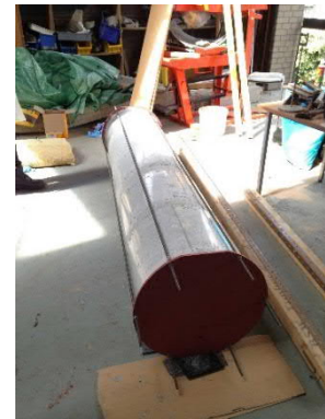
g) Applying permanent post tensioning
