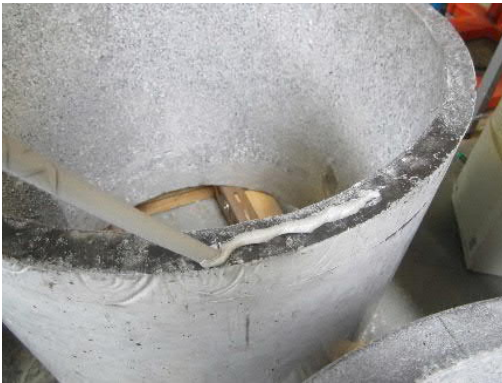
c) Applying epoxy on the both sides
