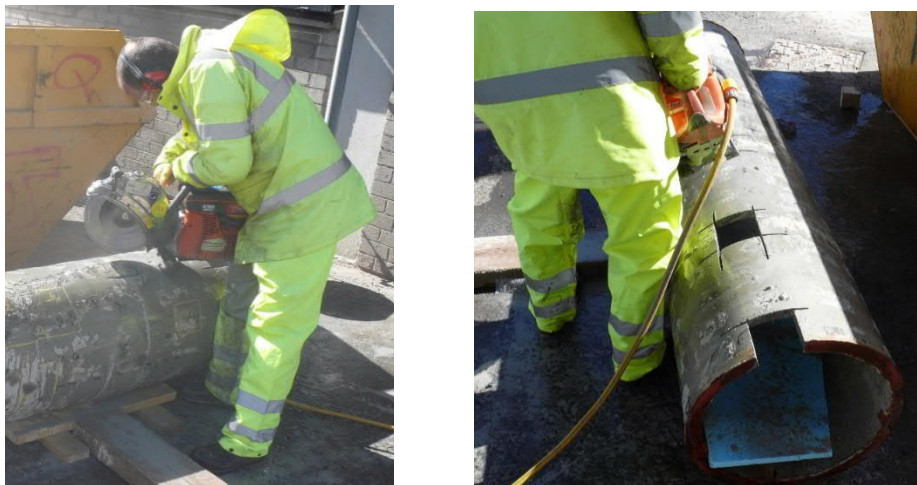
Figure 5.9. Coring of the prototype using the saw
