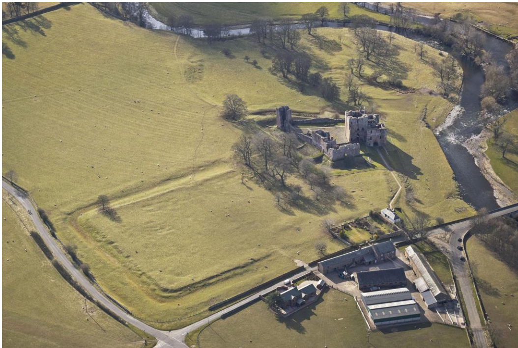
Figure 5.2 - Brougham Castle near Penrith, Cumbria, with the earthwork remains of a Roman camp visible in the lower left as a "shadow site". High aerial photograph by the research-practitioner, 2013.
